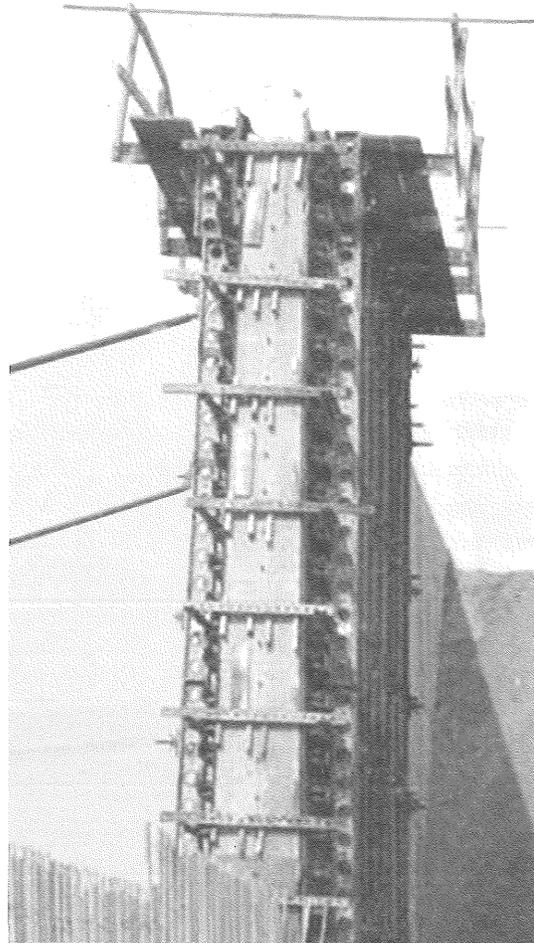
**A specially equipped retaining wall along I-494 continuously sends earth pressure data to the University of Minnesota.**
