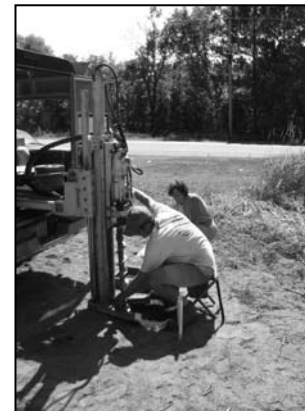
Mechanical coring rig used for MnDOT's deep testing project.
