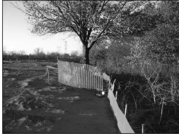
Mound (beneath tree) protected by fence within construction area at Savage Lofts project.
