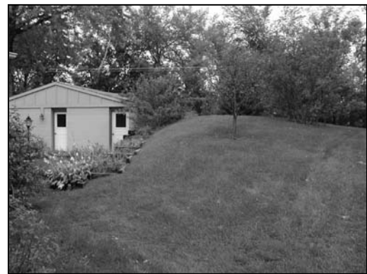
Existing garage built into side of mound at 21HE65.
