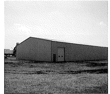
The incubator shell building now partially occupied by Wind Energy Systems
