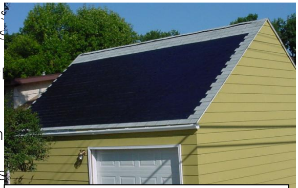
Building integrated solar panels on a Minneapolis garage
