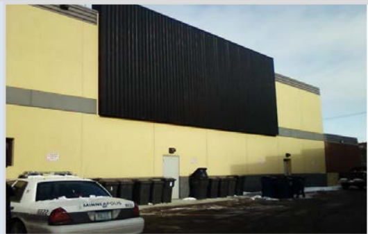
Figure 5. Solar wall on the south side of the 3 rd precinct police station.
