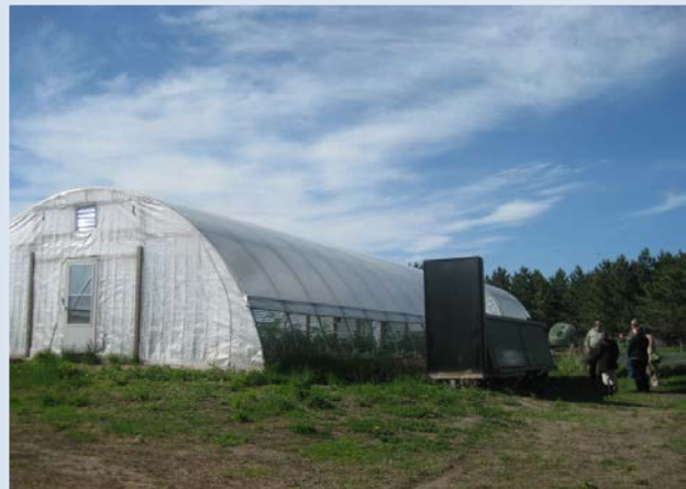
Figure 4. Solar collectors outside of the Flynns' high-tunnel
