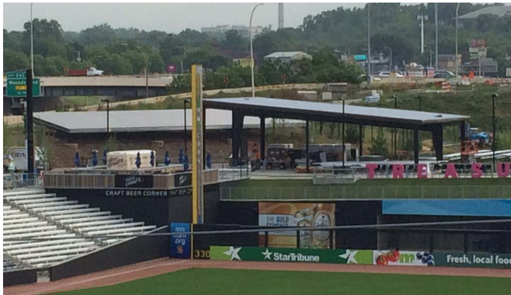
Photo 1: 103.5 kW DC array behind left field at CHS Field in St. Paul
