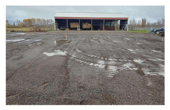
The completed gravel and recycled asphalt pad for the hay bale storage area. (Photo courtesy of the Carlton SWCD)
