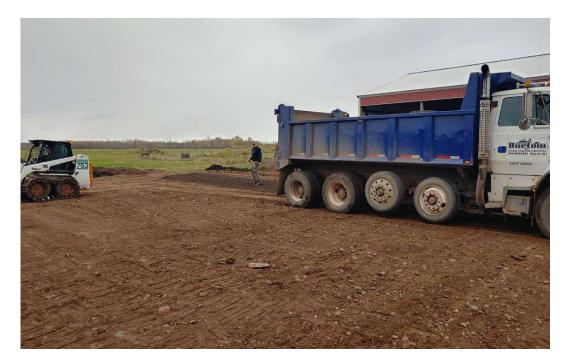
Aravel and recycled asphalt pad is installed for the hay bale storage area. (Photo courtesy of Carlton SWCD)
