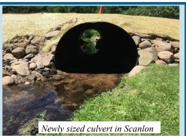
the energy of the water, reduces the wear on the culvert bottom, maintains the culvert elevations, and provides wildlife habitat. In some cases, a flood plain culvert that only flows during very high water may be added, so the stream will have access to the floodplain during a flood event. The bottom line is that a fish friendly culvert will look similar to the stream as it passes under the road.
