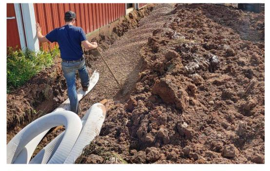
Perforated drain tile is laid in the roof runoff structure's trench to carry clean rainwater from the roof to the stream, thus bypassing the cow yard. (Photo courtesy Carlton SWCD)
